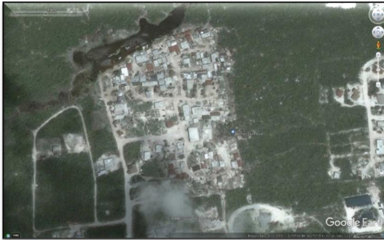
Kat 3 – Santral Dock Yard 2003
