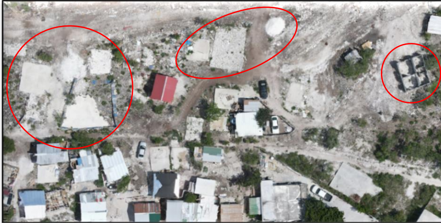
Figure 3 Dock Yard - Evidence of Ongoing Construction
