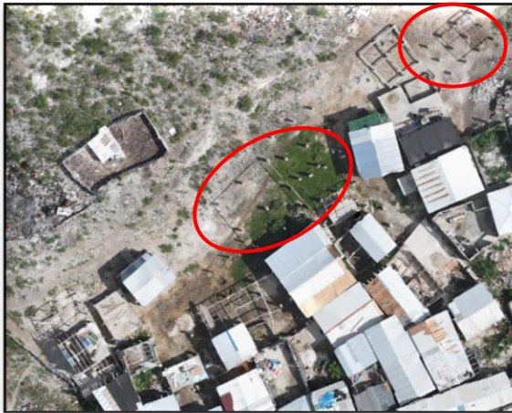
Figure 2 Dock Yard Foundation Stilts
